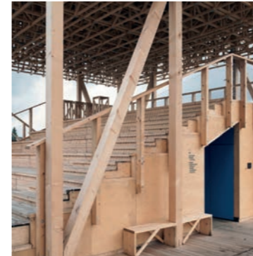
Structure bois - Tom Emerson
