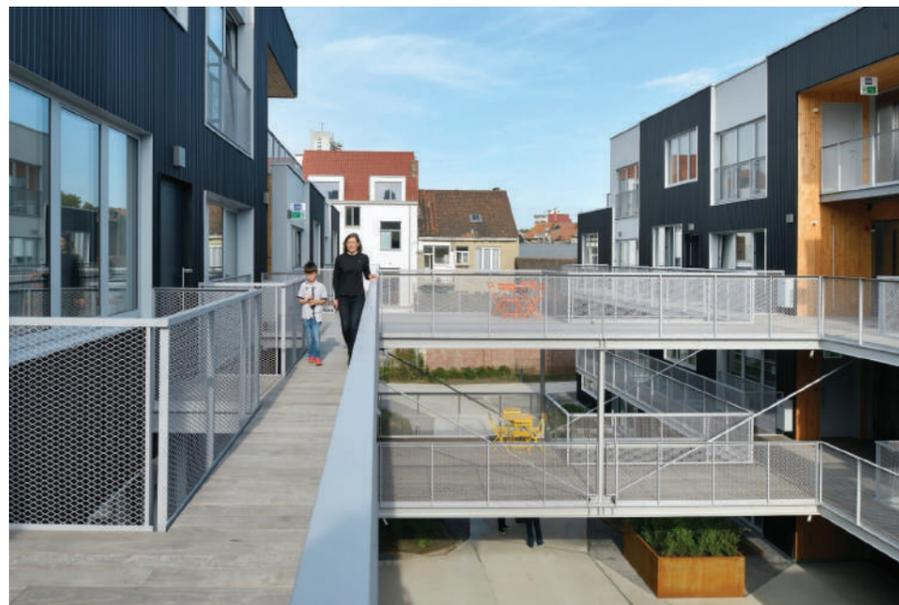
METAL DEPLOYE POUR LES GARDE-CORPS
