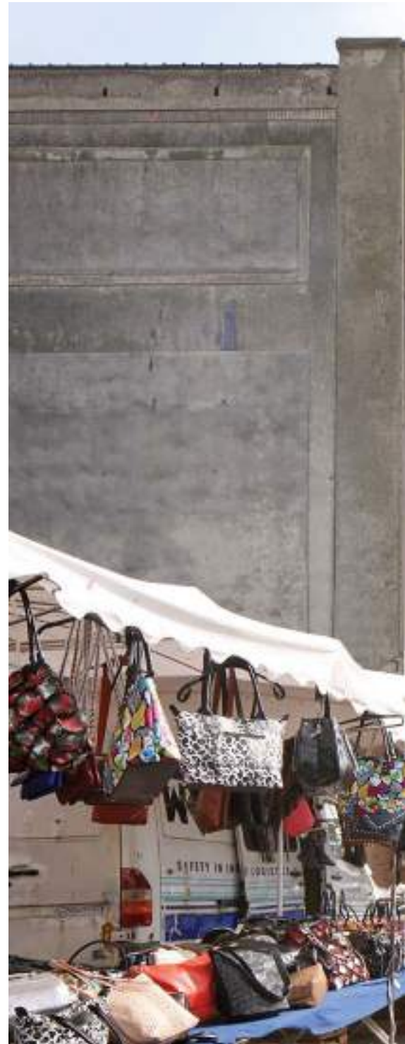
↓ The new construction had to bend itself around the existing Freshmarket, an anonymous warehouse measur- ing around 40 by 50 metres.
