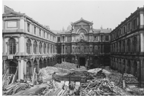
↑ Demolition of the Palais Granvelle
