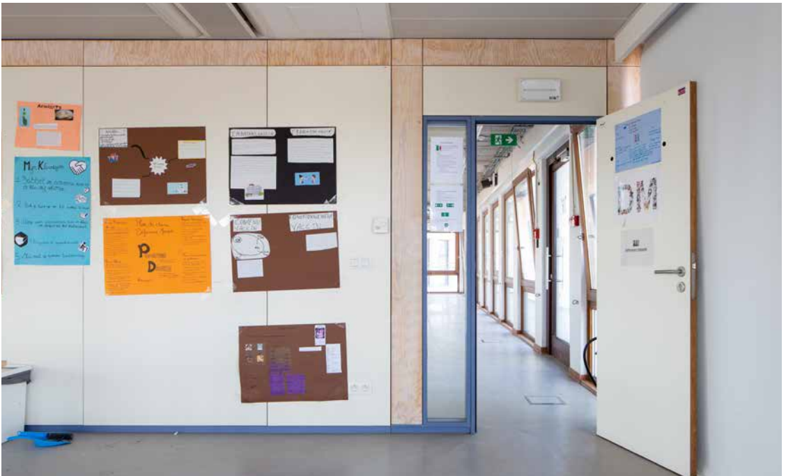
↑ The salvaged partition walls were complemented with wooden panels. Each floor was given a distinct colour for its door frames and baseboards.
