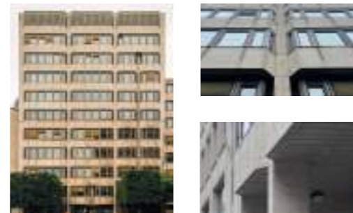
Existing photos, showing architectural character
