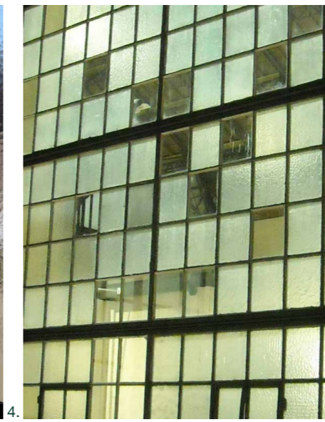
4. ARAT - project Genk C-mine
