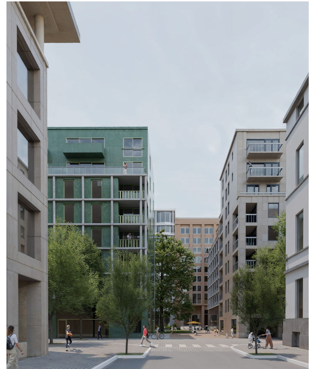
The new passage connects Rue Philippe Le Bon to the garden. Rue Joseph II becomes an active residential street with amenity spaces and entrances at ground floor, and balconies and loggias above.
