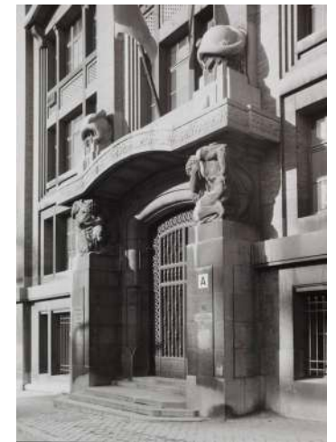
Main entrance with listed framing.
