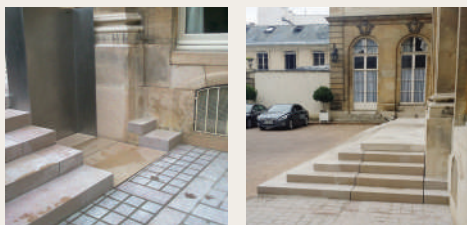
Examples of seamlessly integrated "Stepless" stair lift in heritage project
