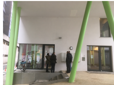
Construction neuve Musin
