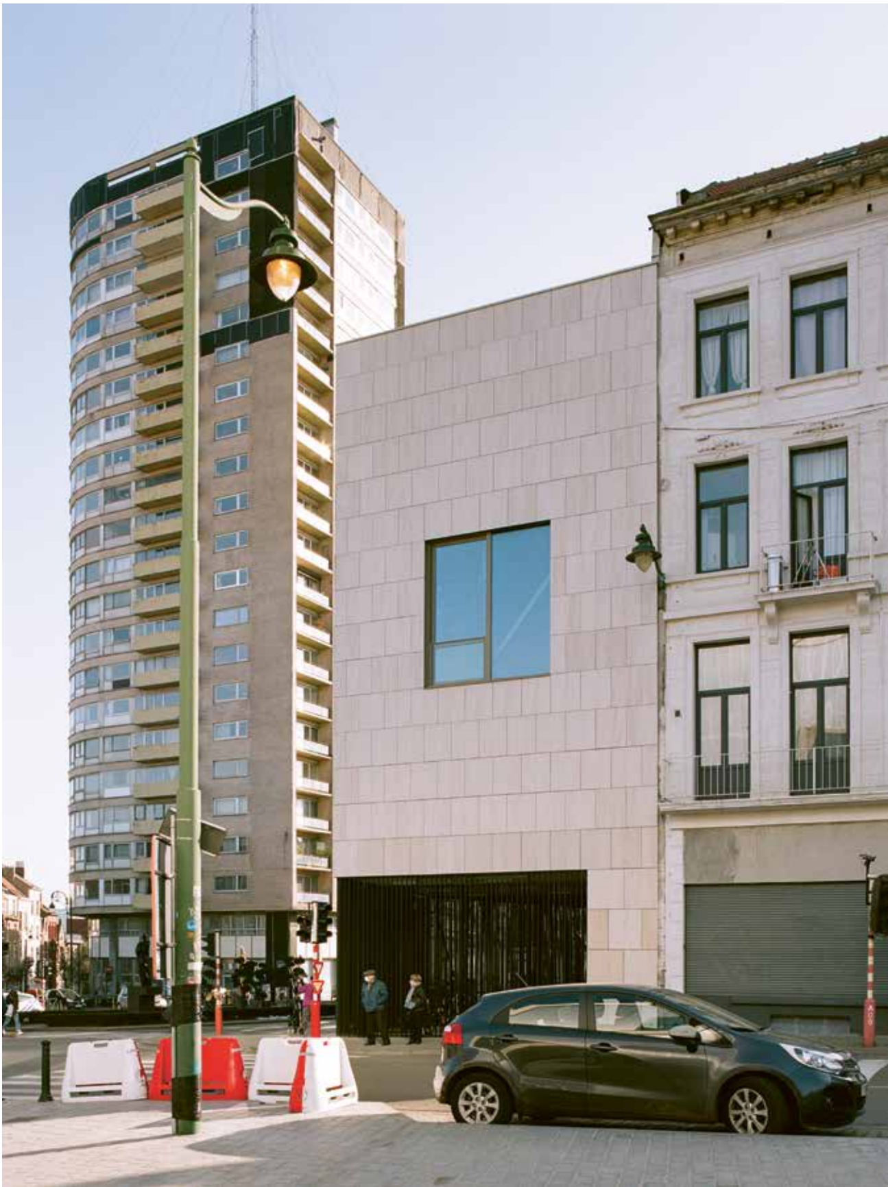
01 The two buildings of the culture and sports complex together form a new link between the municipalities of Forest and Saint-Gilles.
